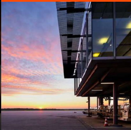
Automated boarding bridges
